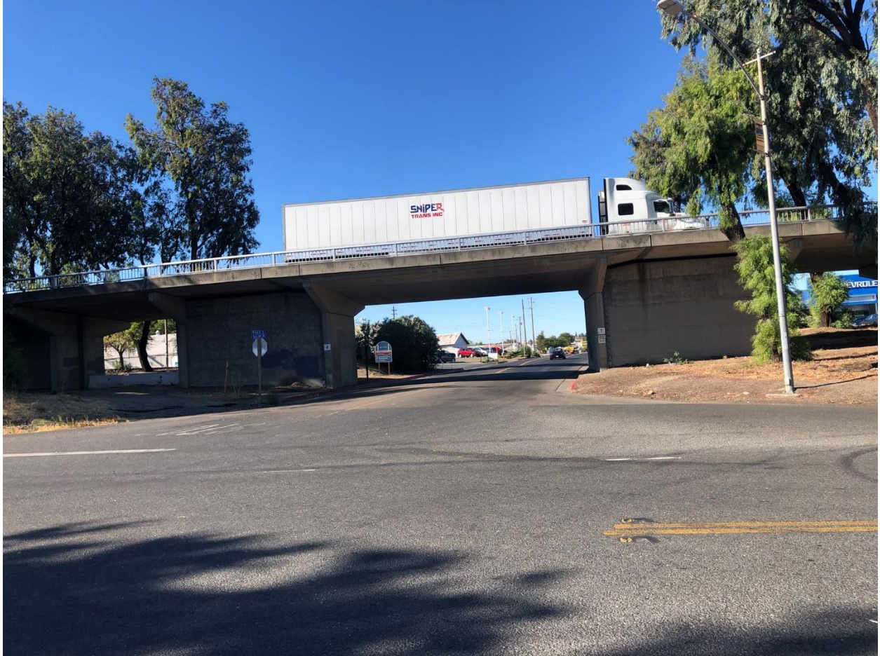
Figure 8: N Front St & SR84, West Approach (1)
