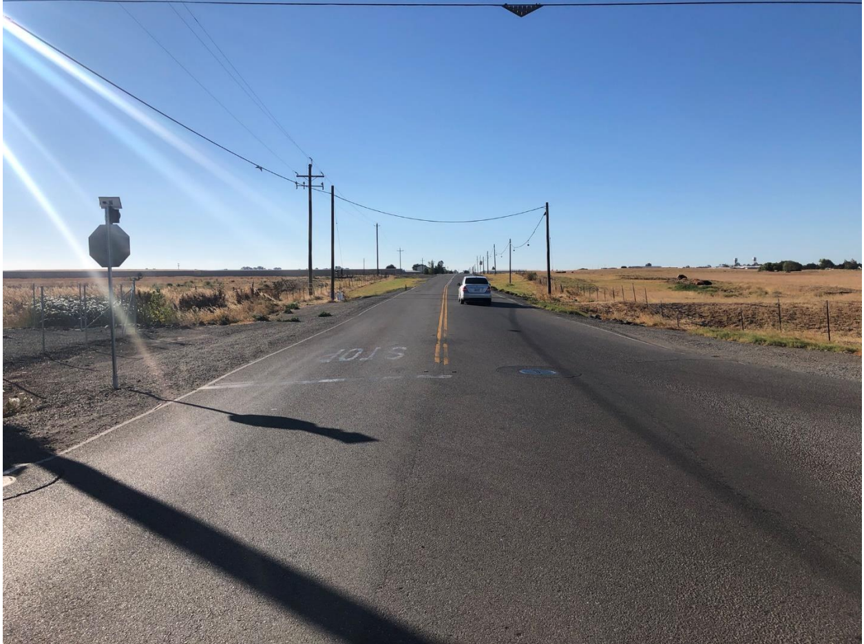
Figure 3: Airport Road and Church Road, South Approach
