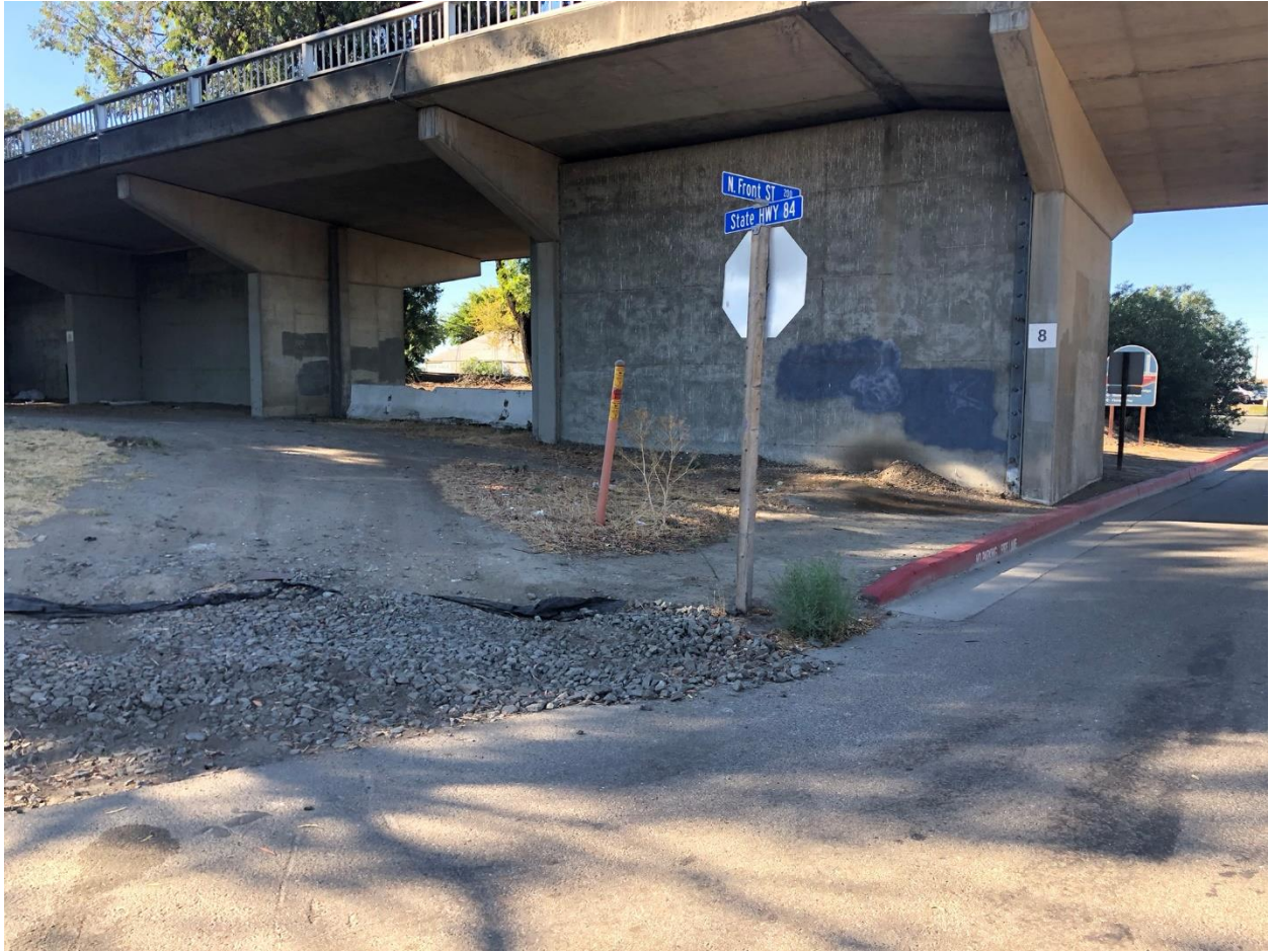
Figure 9: N Front St & SR84, West Approach (2)
