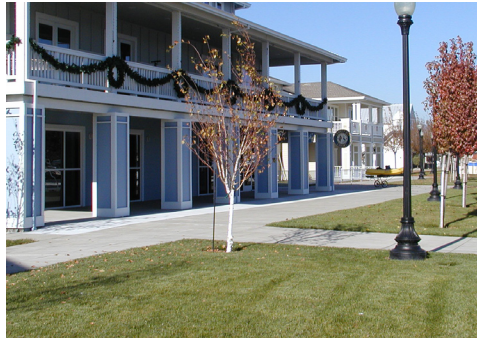
Arcade at Commercial Building
