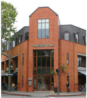
Building sign letters located above corner entrance
