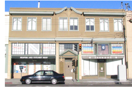
Tile base treatment and transom windows are common to early 20th century commercial architecture
