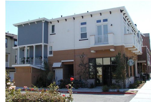
Trash enclosures and service doors are screened from view and incorporate building materials and color
