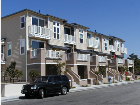
Offset building bays and unique roof forms appear to “break down” the overall building length
