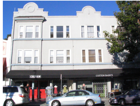
Awnings, upper-story stepbacks and unique parapet add visual interest to the building form
