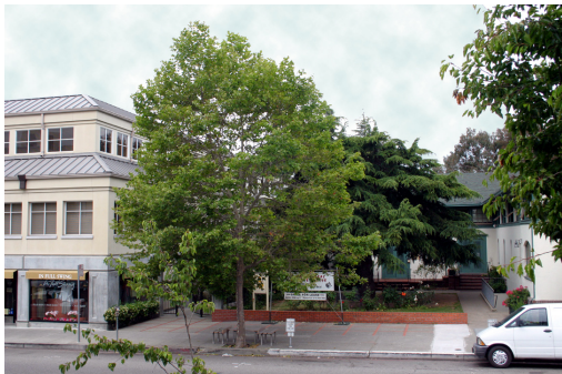
Forecourt utilized by retail, workplace and civic uses
