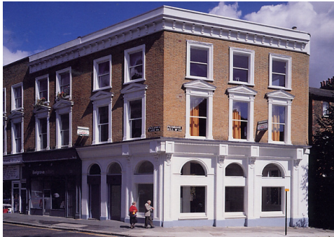
A distinguished building base, cornices and change in materials used to articulate building height
