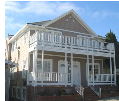
Shared stoop and porch provide gracious setting for multiplex building
