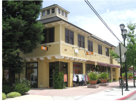
Corner building mass contains unique roof form and shopfront doors
