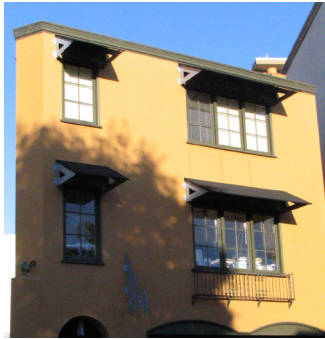
Windows having contemporary shade devices designed to complement building color and materials
