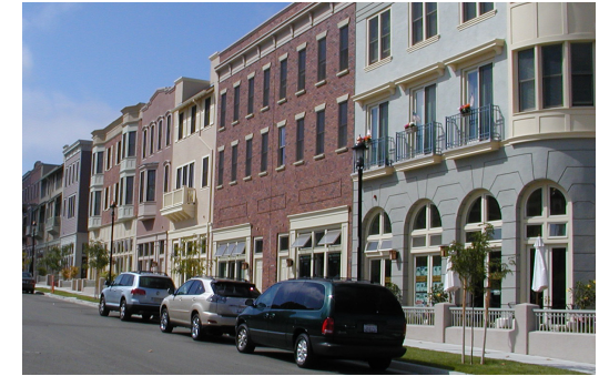
A variety of colors and materials including stucco and brick add visual interest
