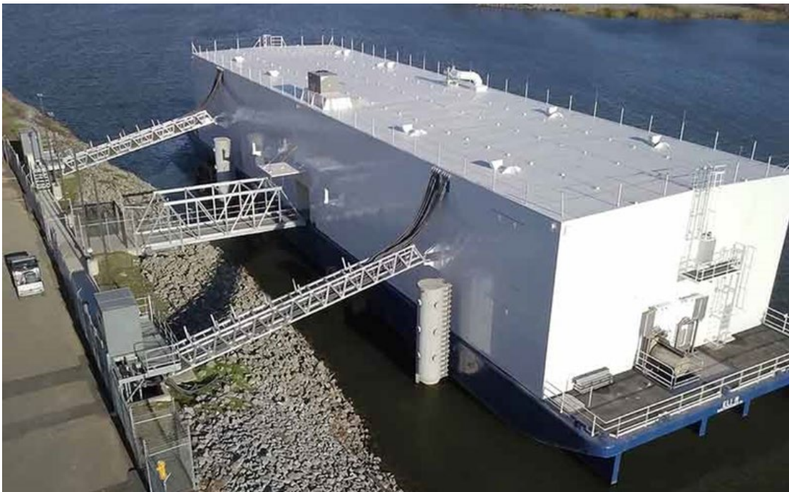
Shown above, the Stockton 1 Data Center, on the San Joaquin River in Stockton, California.
