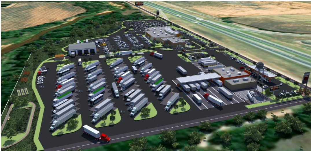
Exhibit P: Shown above, an interstate truck stop design in exploration by SCP’s AEC Creative unit, featuring pull-through overnight spaces (or charging spaces), roadside repair station, and other trucker amenities assuming the transition to driverless / all-electrical will be phased in with new trucking technologies co-existing with traditional truck stop amenities for some period.
