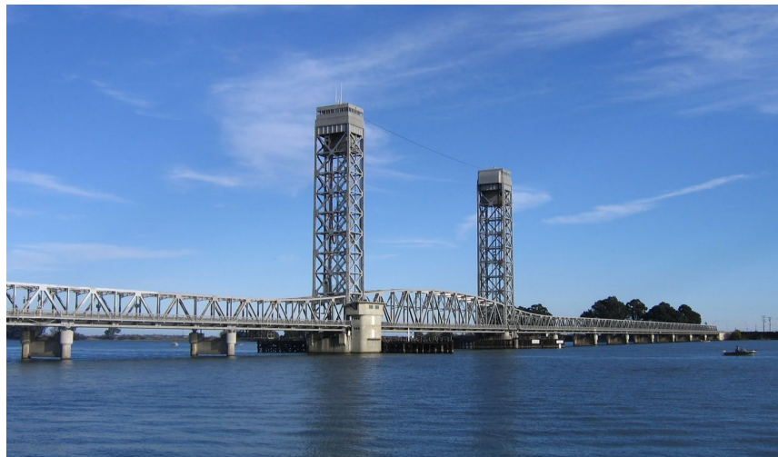
Shown above, Rio Vista Bridge
