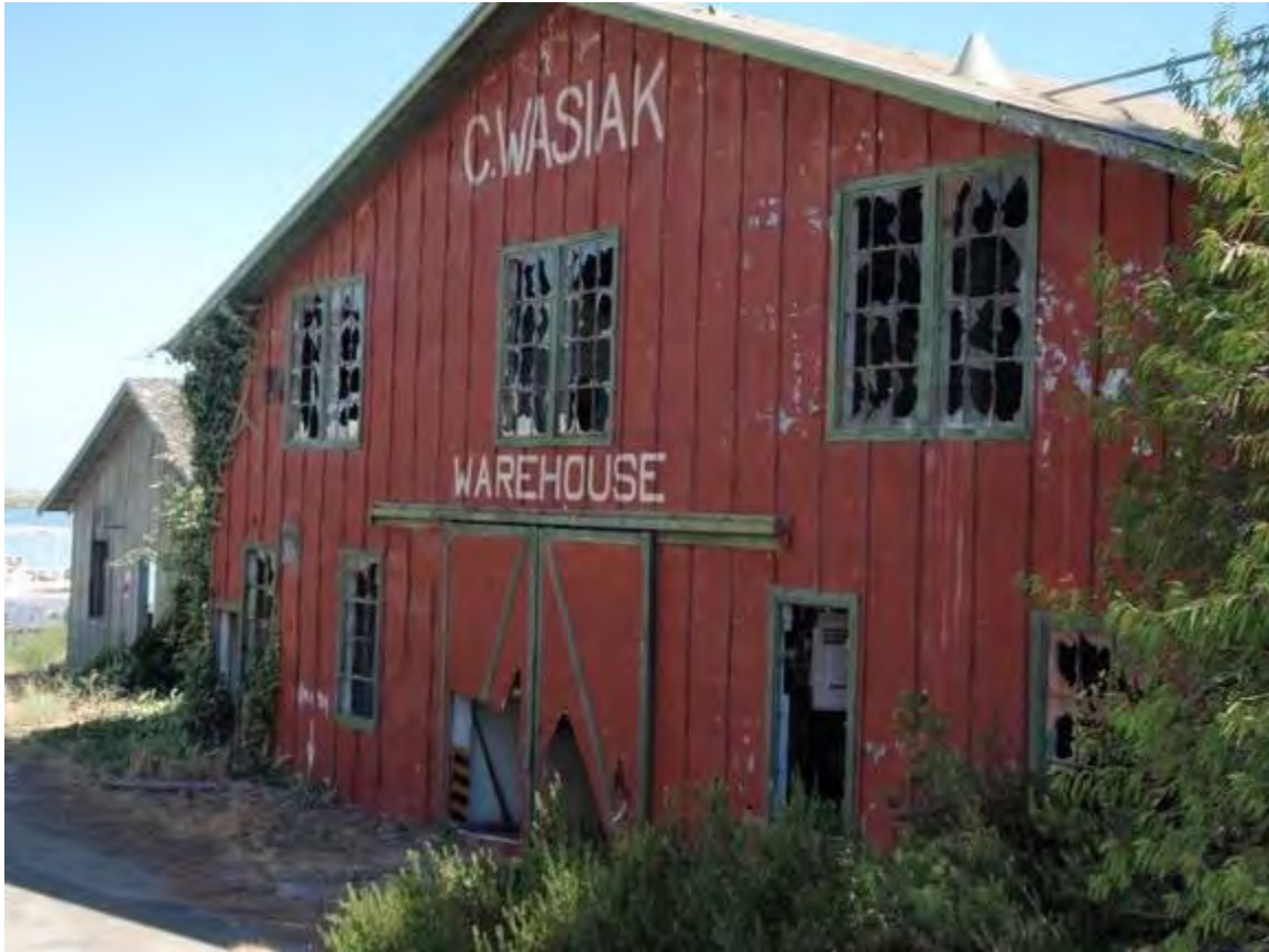
Facility 9: General Purpose Warehouse
