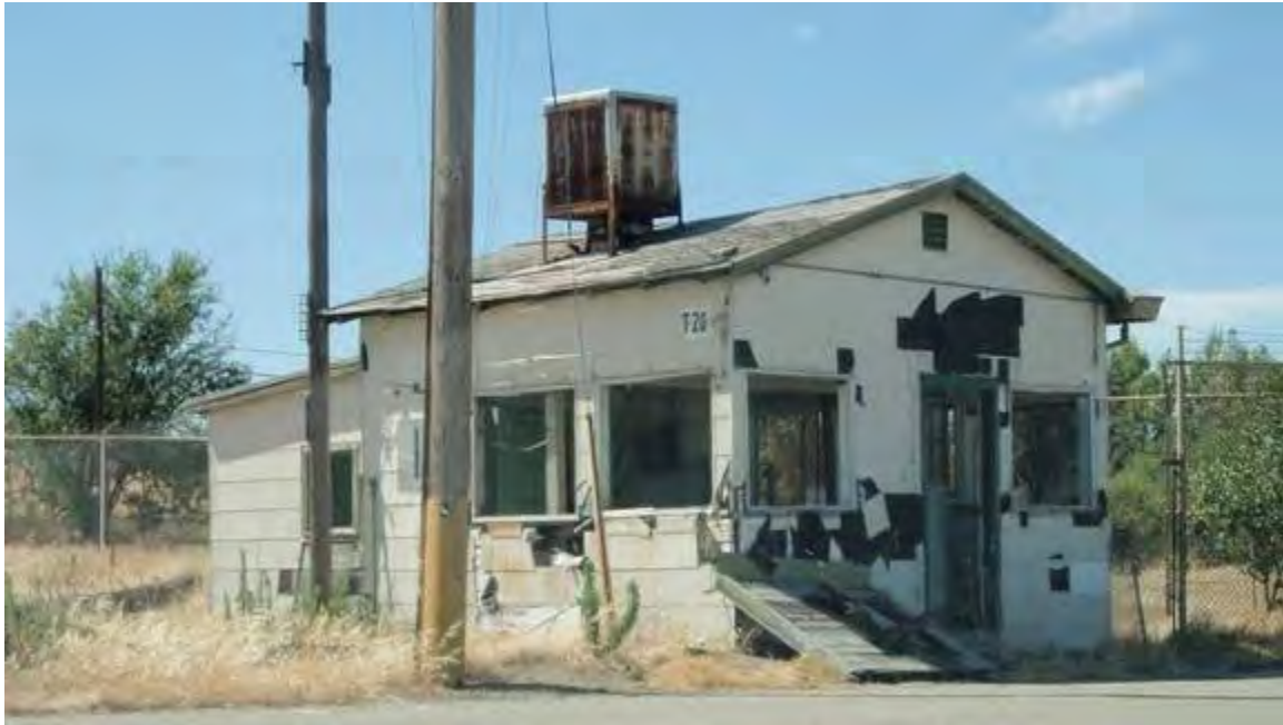
Facility 1: Guard Station
