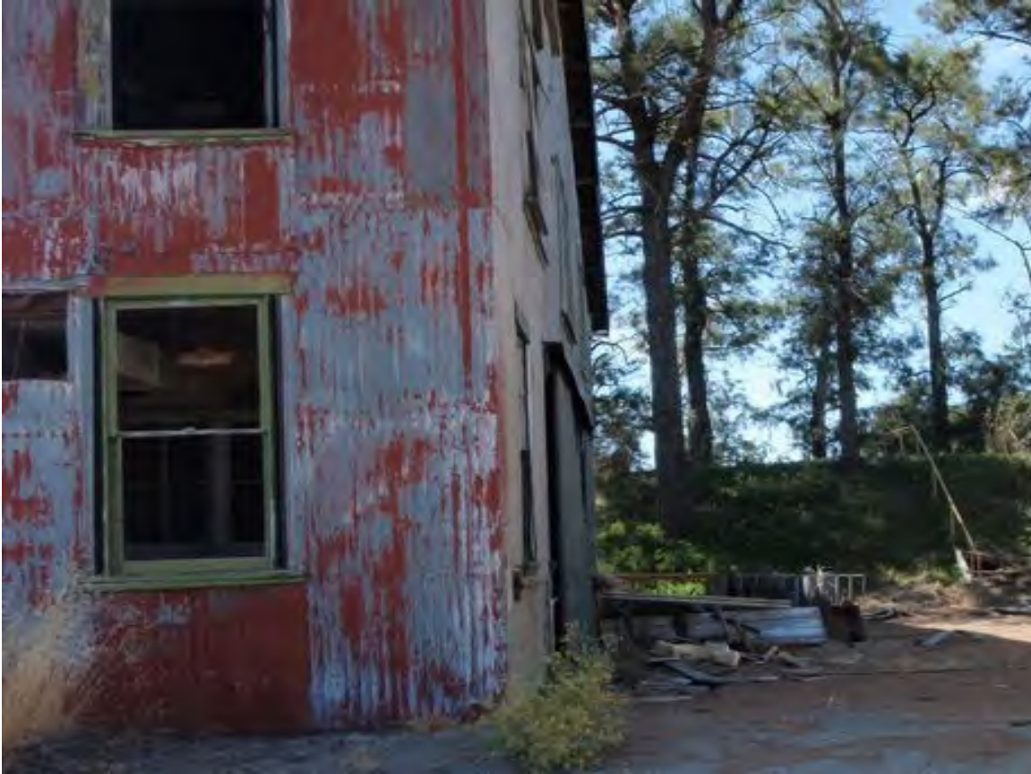
Facility 8: General Purpose Warehouse
