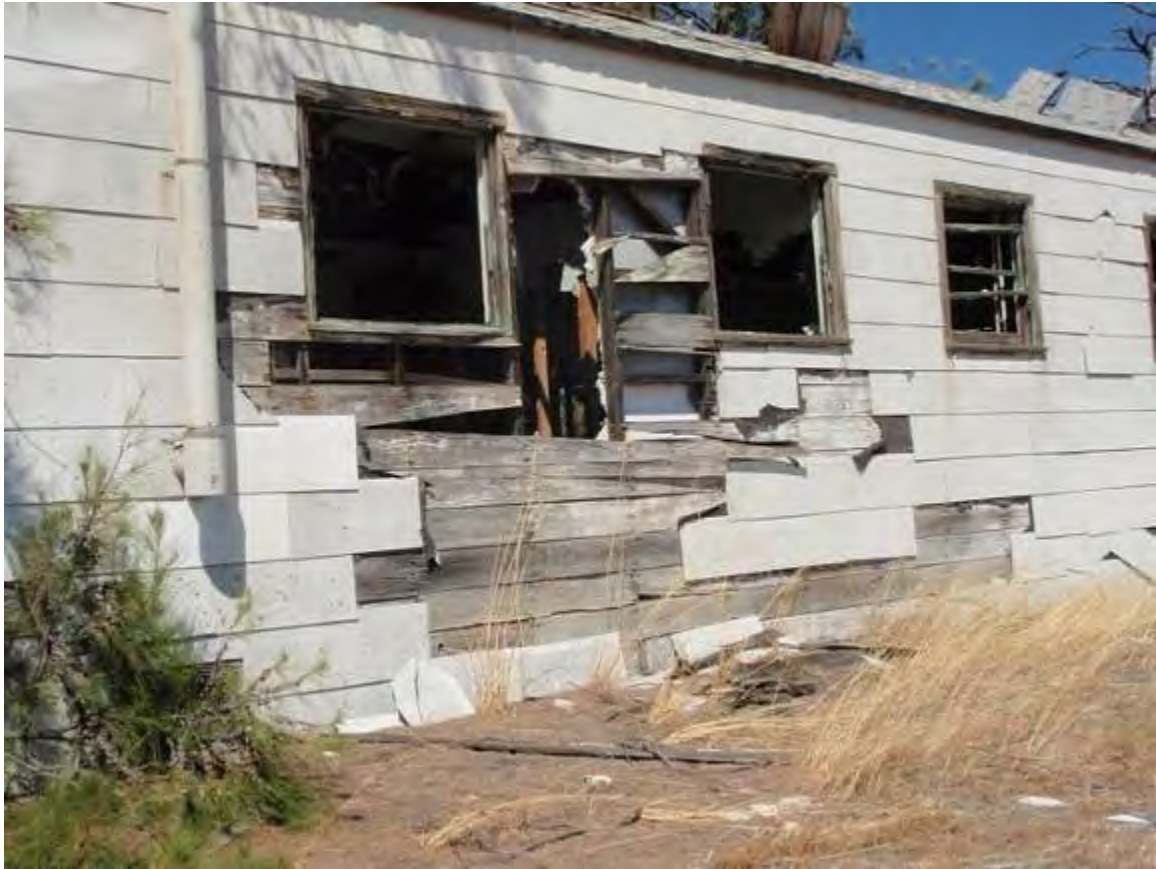
Facility 12: Administration, Enlisted Barracks
