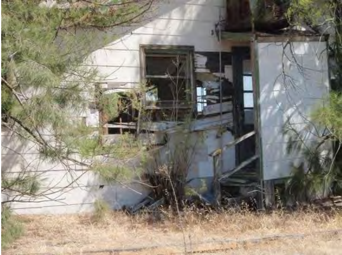
Facility 12: Administration, Enlisted Barracks
