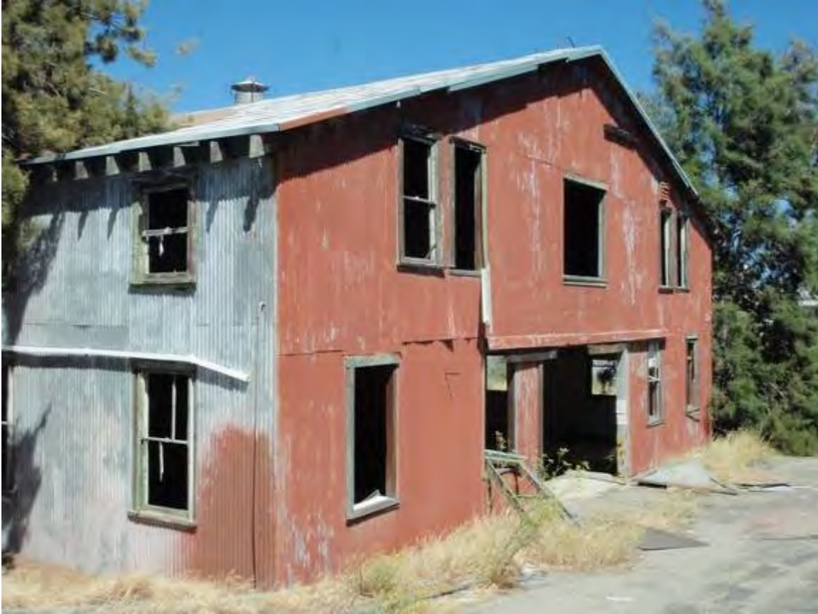
Facility 8: General Purpose Warehouse
