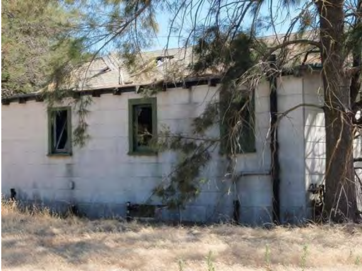
Facility 12: Administration, Enlisted Barracks
