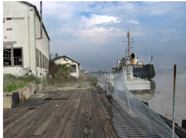
Photo 10. Looking north. S-103 and S-102 Ship repair docks.
