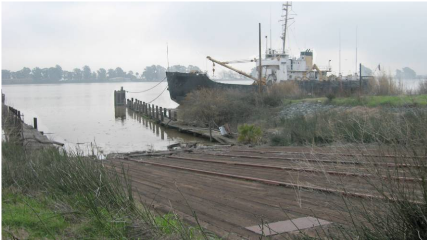
Photo3. Looking west. S-100 Marine railway ramp where boats were drawn out of the river for repair. Boat cradle and winch house were removed. Emergent wetlands along edges of ramp.
